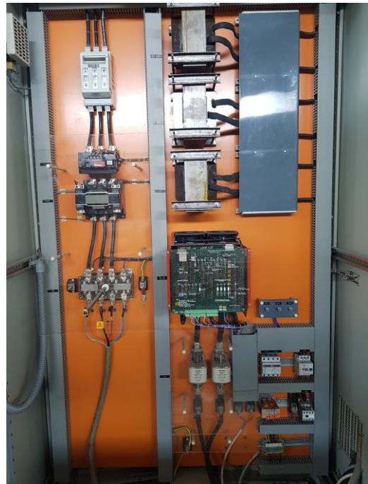
Regular Wave Generator Controller Controls the generation of the regular waves
